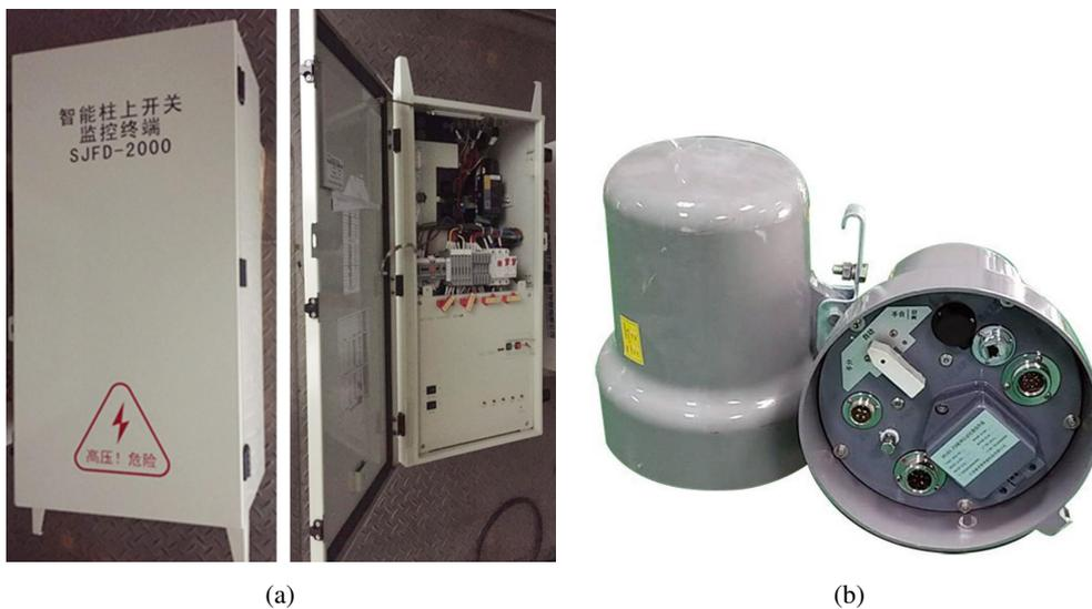
Fig. 7. The appearance and interior of the typical FTUs in the field: (a) the first type; (b) the second type
