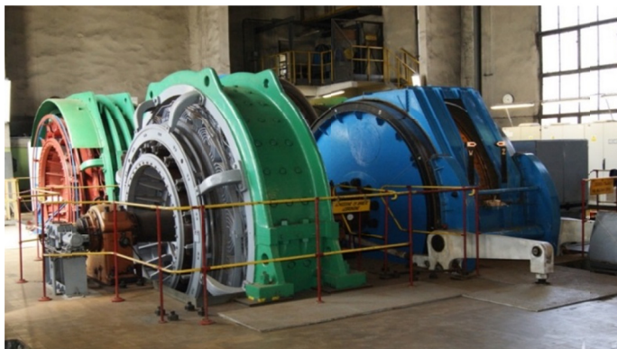
Fig. 1. The Andrzej V East shaft braking system
