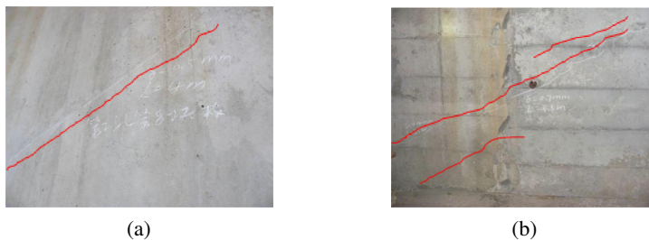
Fig. 4. Cracks distribution on the web: (a) Crack on the No. 8 block exterior surface ( L = 4 m, \delta = 0.5 mm, \alpha = 45^\circ ); (b) Interior surface oblique crack ( L = 8 m, \delta = 0.5 mm, \alpha = 35^\circ )
