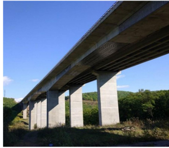
Fig. 1. General view of the rehabilitated highway bridge
