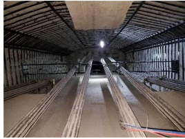
Fig. 9. On-site installation of external prestressing tendon
