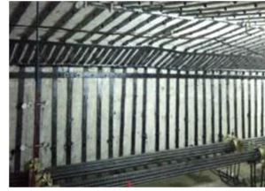
Fig. 10. Steel plates on the interior of the girder web
