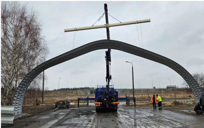
Fig. 7. Assembly of group of UBM panels
