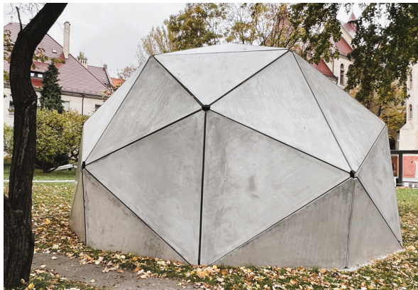
Fig. 1. Panel shell mock-up in geodesic dome (Fuller's dome) geometry completed as part of the ReSa project (Author's photo)
