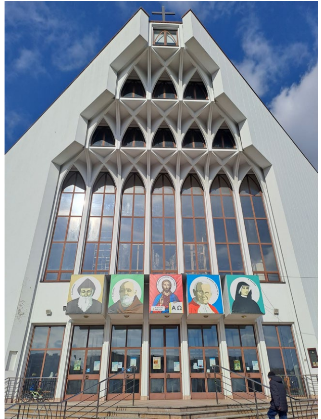
III. 4. St Brother Albert Church in Czyżyny — detail of the front facade. Photo by the Authors.
