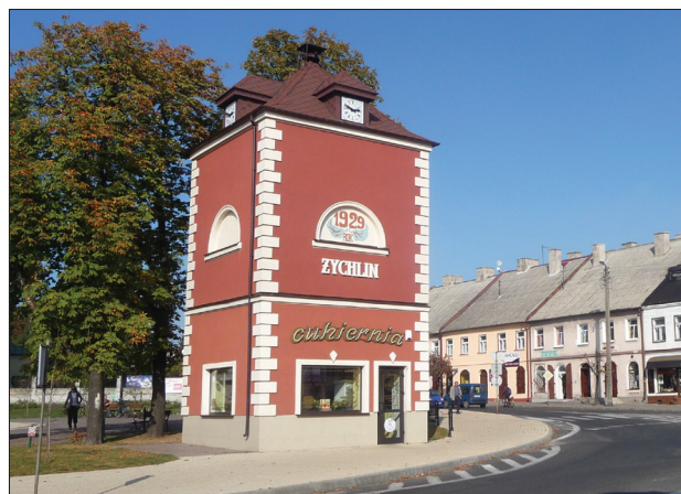
9. Stacja transformatorowa z zegarem wybudowana w 1929 r. na osi ul. Narutowicza, stan obecny. Fot. autor, 2015 9. Transformer station with a clock erected in 1929 on the axis of Narutowicza Street before it joins 29 Listopada Square (former Market Square) – today. Photo by the author, 2015
