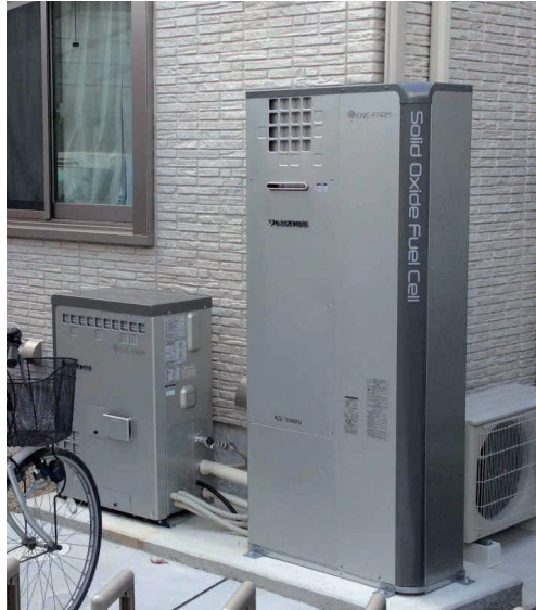
Figure 5. Small scale SOFC 700 W “ENE-FARM” Type S (ENE-FARM installed 120 000 residential fuel cell units in Japan)
