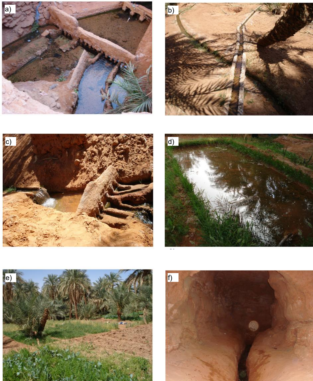
Photo 1. The different parts of a foggaras: a) The main kasria of El Meghaier foggara in the oasis of Timimoun; b) Seguias of El Meghaier foggara to bring water until Madjen in the oasis of Timimoun; c) Secondary kasria of La Salma foggara in the oasis of Timimoun; d) Madjen (tank) of La Salma foggara in the oasis of Timimoun; e) Guemoun (garden) in the oasis of Timimoun; f) A section of the non-active part of the gallery of the foggara of La Salma (phot. B. Remini)
