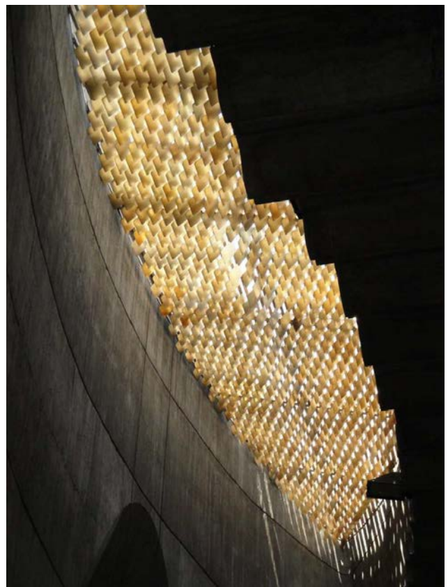
Fig. 5. Rooflight above the presbytery.
