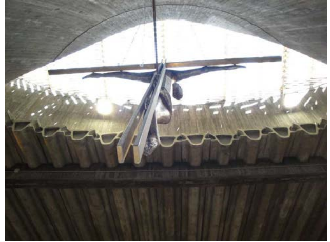
Fig. 4. Rooflight and bone-beams .
