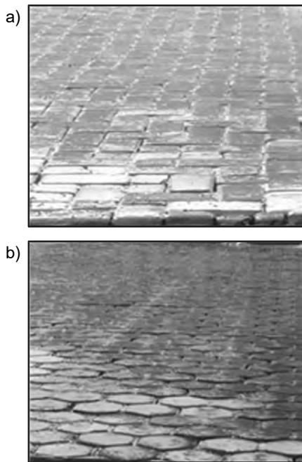
Photo 3. Paving blocks: a) rectangular, b) hexagonal
