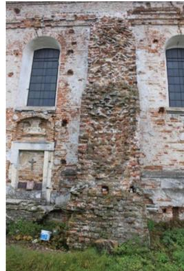
Fig. 9. A damaged abutment.
