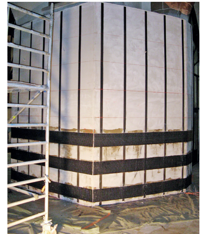
Fig. 14. CFRP-constraining strips around column base during execution
