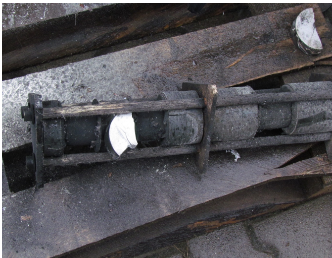
Fig. 5. Fastening elements and damaged varistors following the unsealing, breakdown and fire of an HV surge arrester
