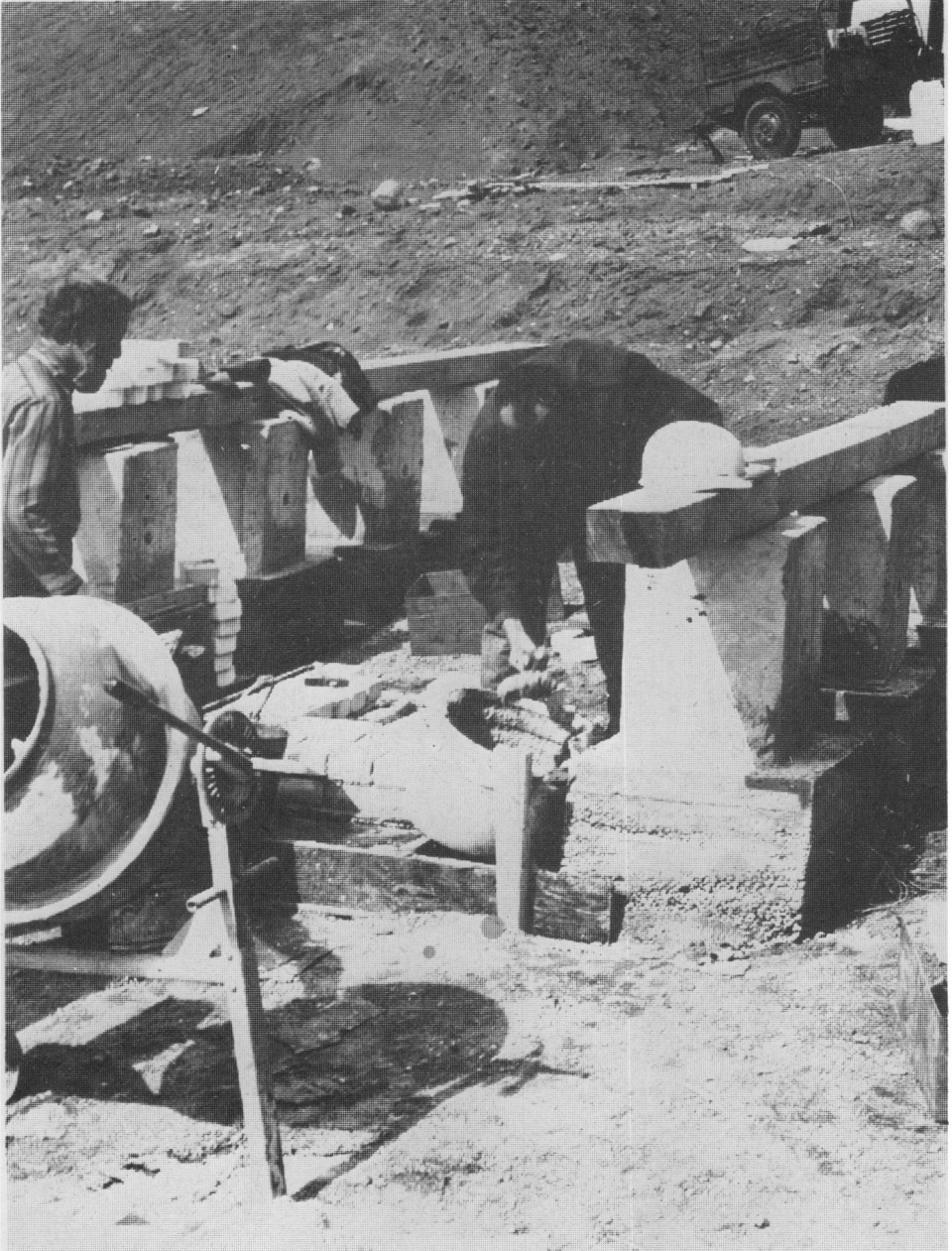
Fig. 4. Foundations of magnetic pavilions under construction
