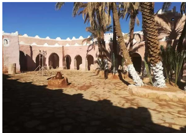
Photo 2. Placette of Nouaday for sharing foggara waters; phot. Ch. Rezzoug
