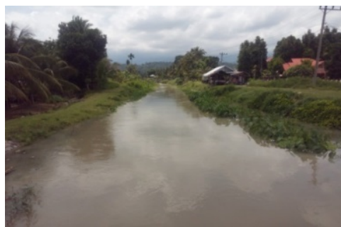
Photo 1. The condition of the structure, the primary channels of Baro Kanan (phot. A. Azmeri)
