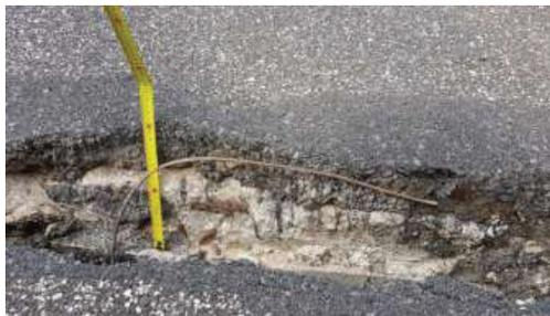
Fig. 7. Bridge Deck, Asphalt pavement and cement concrete deck thickness at the 88 mjoint .
