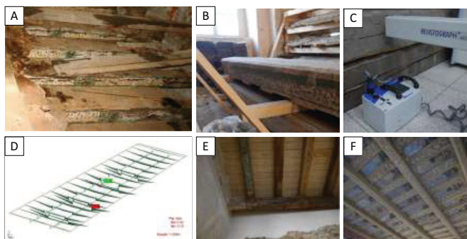
Fig. 2. Recovery of timber structural beams
