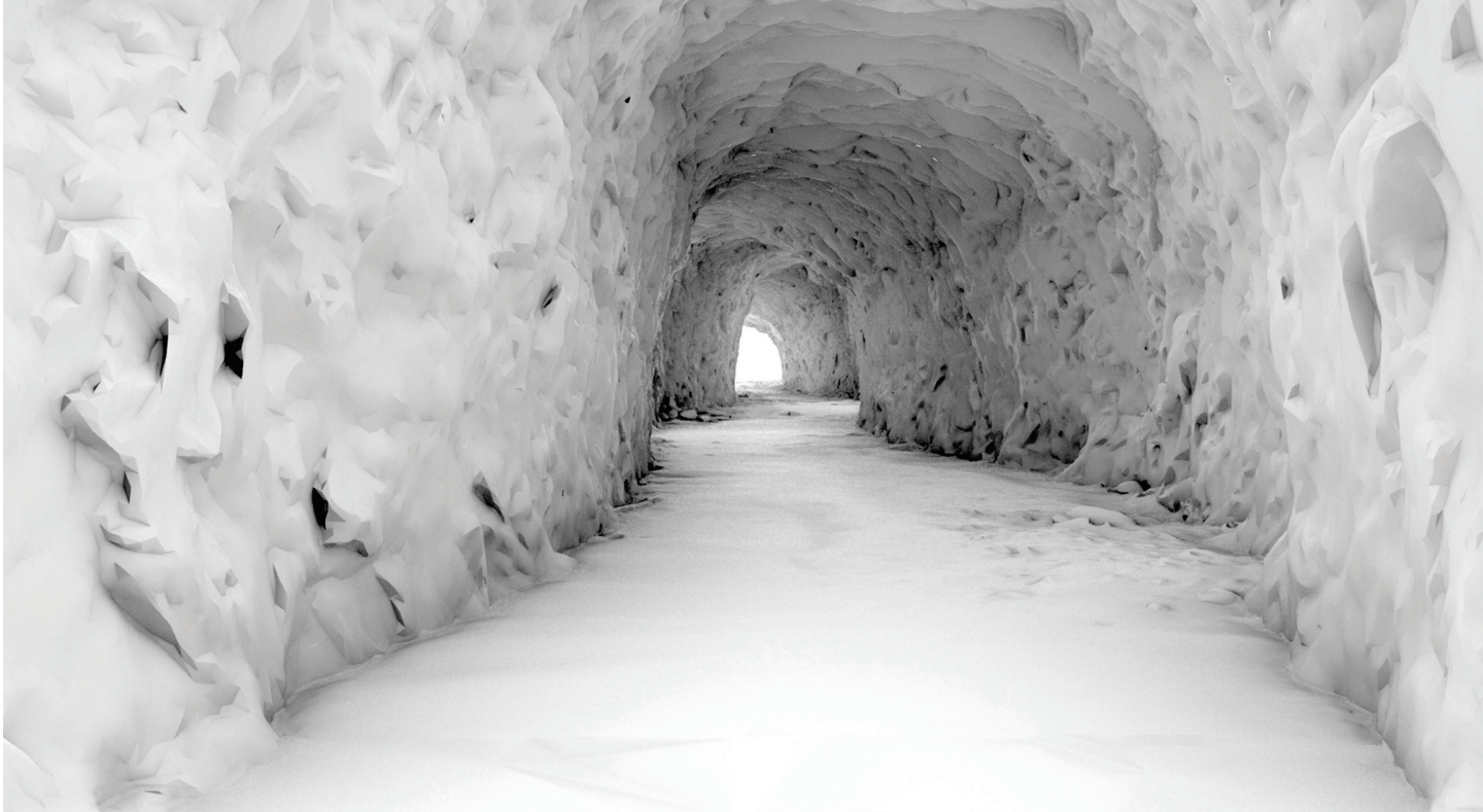
Fig. 6 A view into a rock-blasted unlined hydropower tunnel investigated in the Tunnelroughness project
