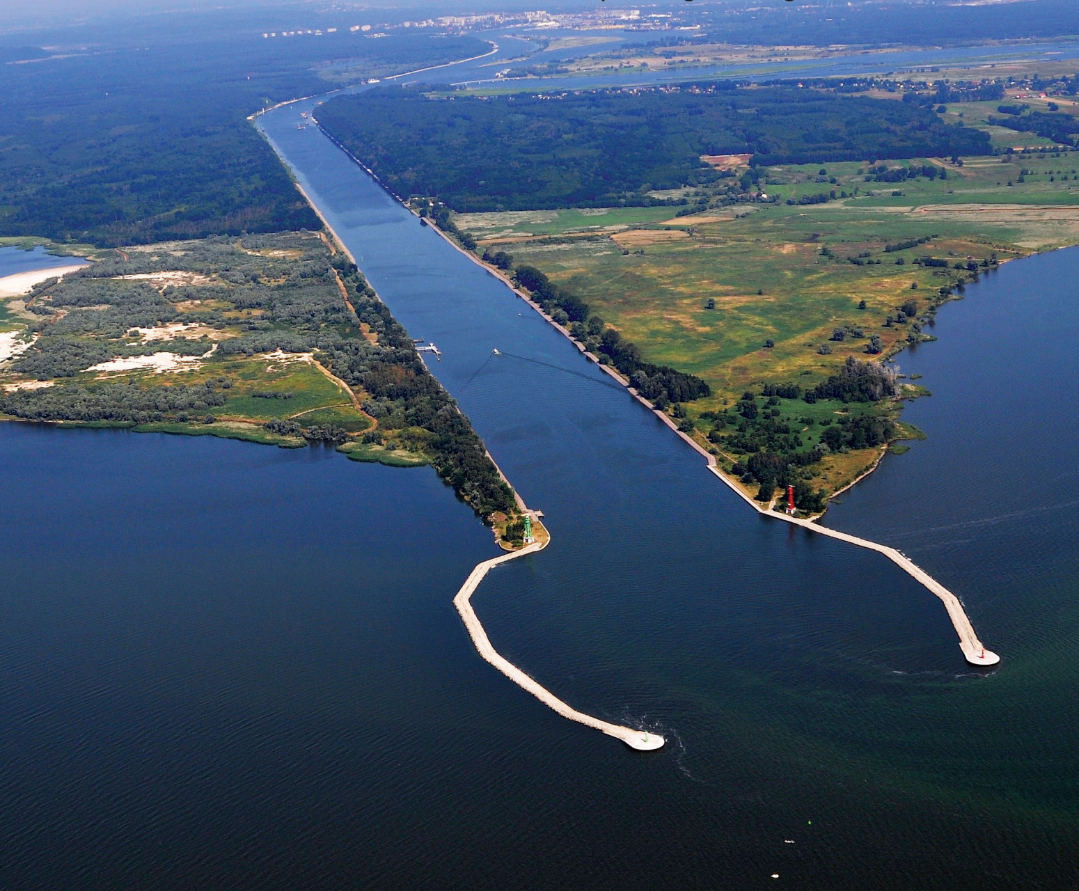
Fairway Gate 1 where the Świna River enters the Szczecin Lagoon. Aerial photograph after completion of the construction process
