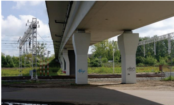
Fig. 2 Inspected bridge pier
