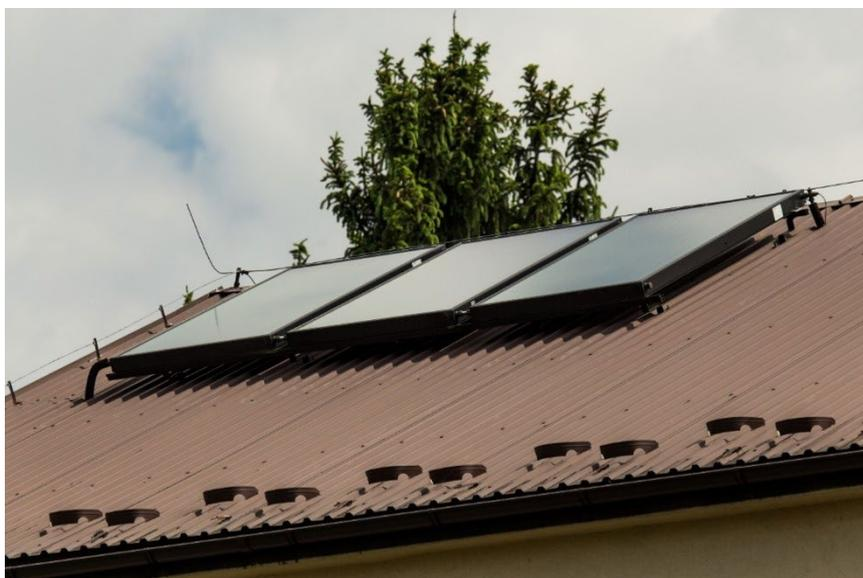
Fig. 1. The flat plate collector installation in detached house
