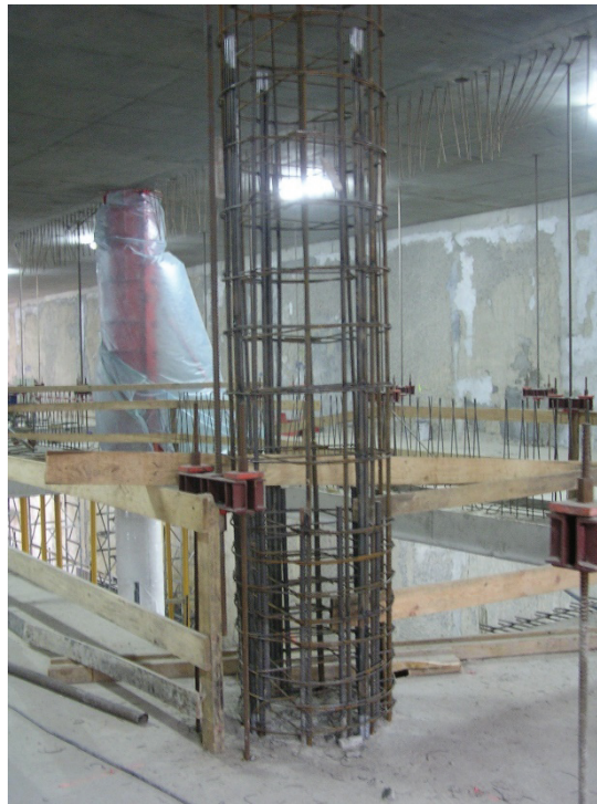
Fig. 4. The column reinforcement, concreted through an opening in the slab [1]
