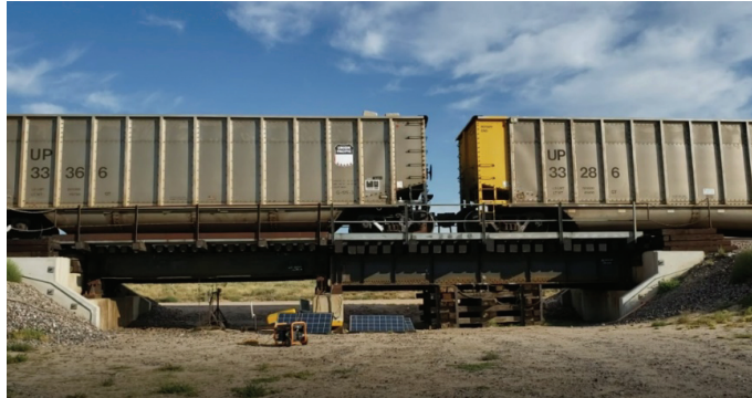
Fig. 3. The West Steel Bridge
