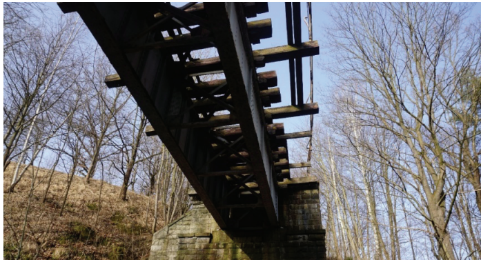
Fig. 1. A typical riveted DPG spans with an open deck (no ballast)
