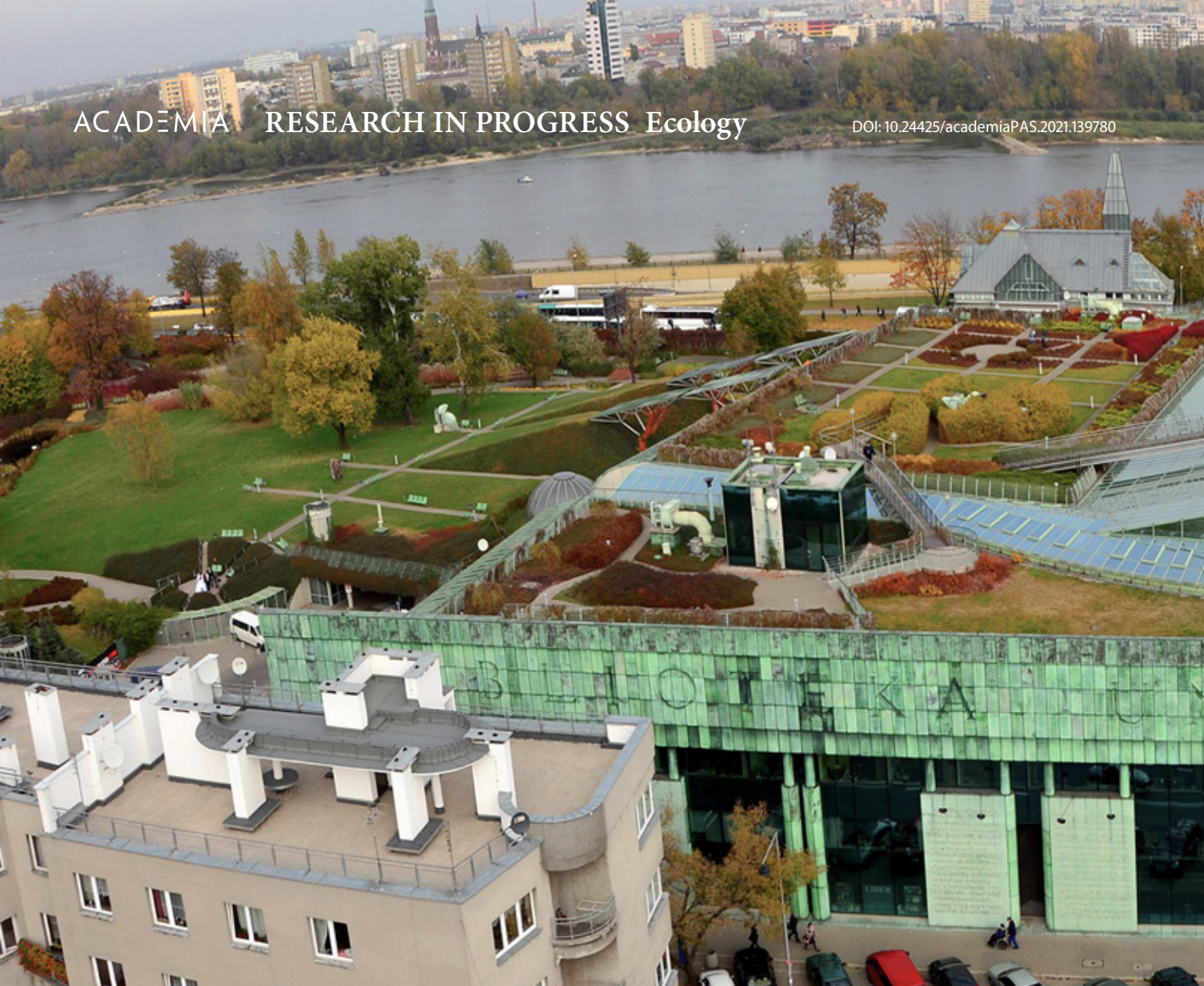
Rooftop garden of the Warsaw University Library building
