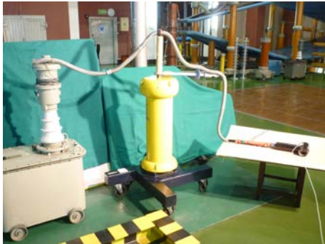
Fig. 1. General view of the testing setup (the MV transformer and the voltage divider).
