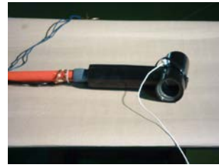
Fig. 3. View of the investigated T-type connector with a fastened AE sensor.
