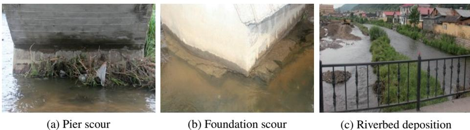
Fig. 4. Main damages of substructure
