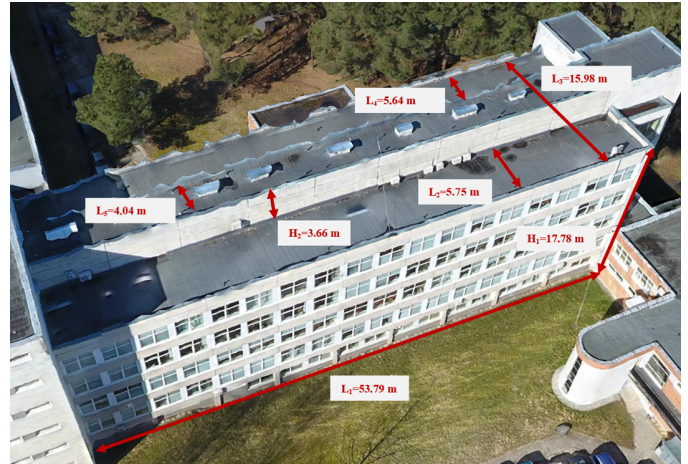
Fig. 9. Linear take-offs of the roof and façade on the basis of the photogrammetry model (source: own study)
