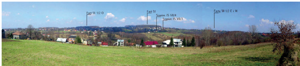
Ill. 6. Panorama of the group of Fort 51 'Rajsko' as viewed from the foreground. A clearly visible function of the green masking, stretching and blurring the silhouette of the fort (deforming and disinforming effect). On the left side of the trees of Fort 51 'Rajsko', a thinner side mask is clearly visible. Photo by P. Leonowicz.
