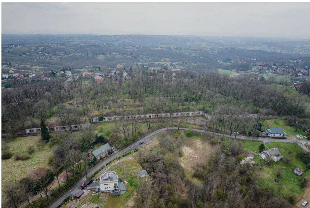
Ill. 4. Aerial view of Fort 51 'Rajsko'. Photo by J. Gawron.
