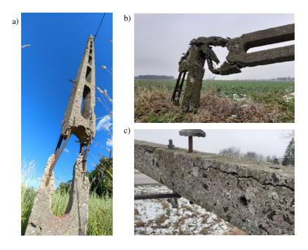
Fig. 6. View of the damaged pole (a); Extensive detachment reinforcement cover in the element (b); Destruction of the element (c)
