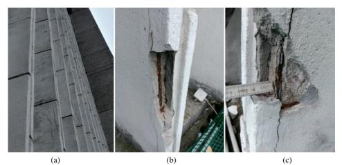
Fig. 5. View of extensive damage to façade elements (a); Example of element chipping (b); Measurement of carbonation depth and lagging (c)
