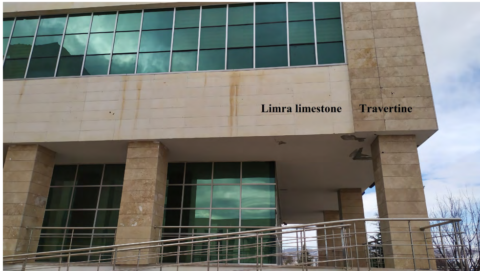
Fig. 1. View of a building where limra limestone and travertine are used as exterior cladding (Kırşehir Ahi Evran University)
