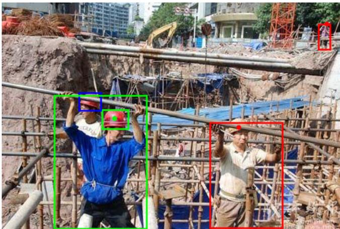
(c) failure to detect both person and hard hat due to occlusion
