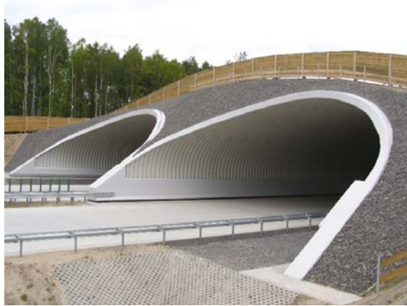
Fig. 1. Crossing for animals over a road constructed as the SSCS
