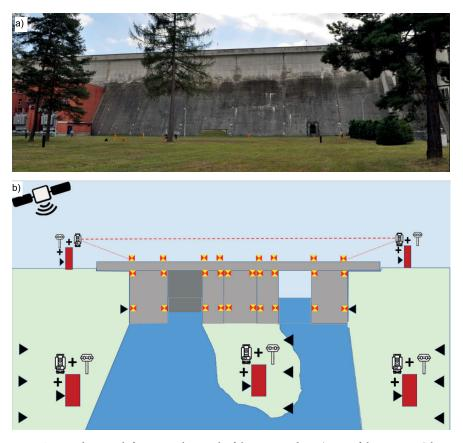
**Fig. 6.** Suggested approach for a control network of the concrete dam: a) view of the structure (photo taken from the island: location of the middle pole in the draft), b) draft of the fundamental alterations in the geometry and infrastructure of the control network; source: own elaboration, phot.: *J. Zaczek-Peplinska*
