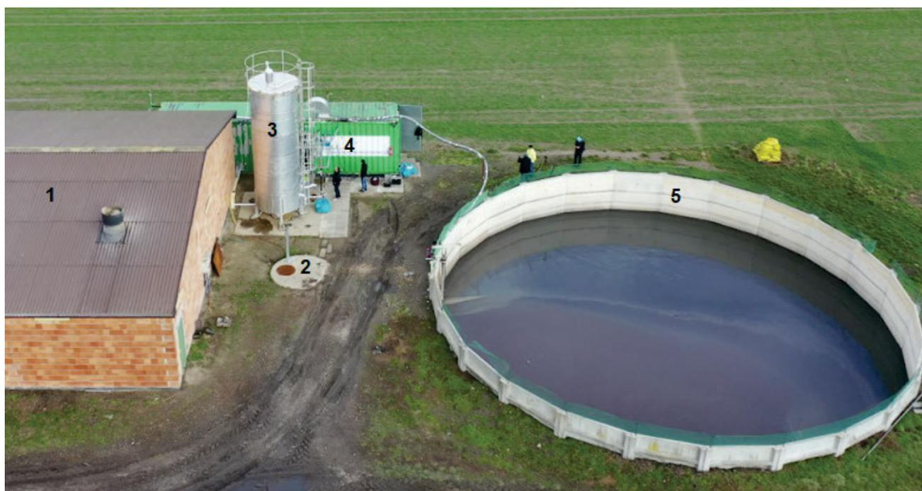
**Fig. 1.** Mobile pilot installation, example of the location of an agricultural biogas plant on a farm; 1 = livestock building, 2 = manhole to the well, the so-called “pre-tank for pig slurry”, 3 = digester, 4 = container with the installation, 5 = digestate tank the so-called “lagoon”; source: own elaboration
