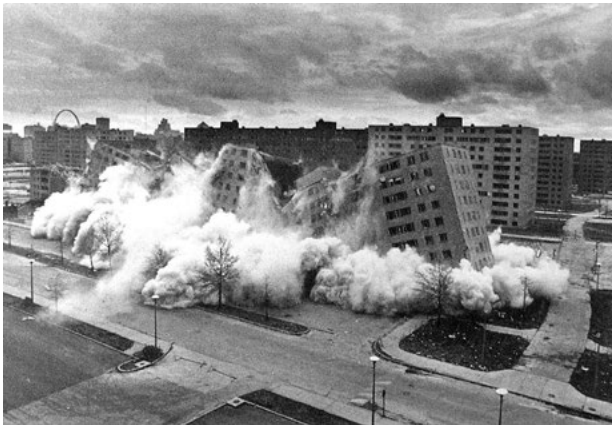
Il. 8. The spectacular moment of the demolition of the Pruitt-Igoe development in 1972, which was built in St. Louis in 1955. Source: Roger Trancik, Finding Lost Space, Theories of Urban Design , New York 1986
