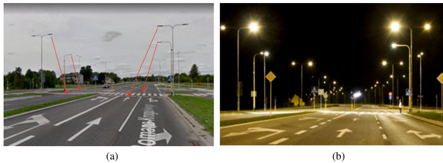
Fig. 4. Daytime view of pedestrian crossing no. 4 with dedicated pedestrian crossing lighting on a sectional two-lane and three-lane two-way street with street lighting on both sides (a) and the visibility of a pedestrian in light-colored clothing waiting to cross the street (b)
