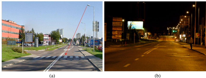
Fig. 1. Daytime view of pedestrian crossing no. 1 without dedicated lighting located on a two-way single-lane street with street lighting located only on one side (a) and nighttime visibility of a pedestrian in light-colored clothing waiting to cross the street (b)
