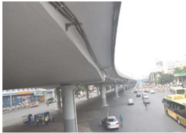
Fig. 1. Actual view of the elevated bridge
