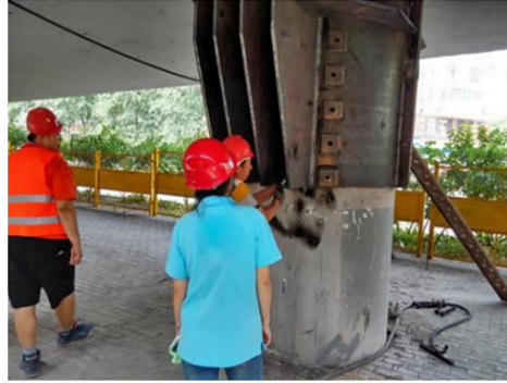
Fig. 11. Reinforcement with hoop bars
