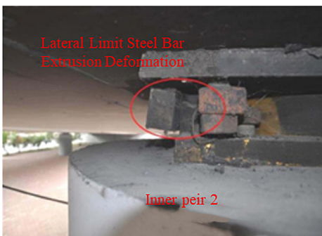
Fig. 6. Lateral limiting steel bar under compression deformation
