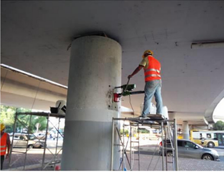
Fig. 10. Pier column drilling
