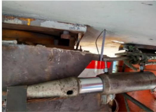
Fig. 12. Prestressing of hoop bars
