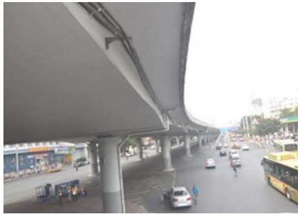
Fig. 1. Aerial view of the elevated bridge
