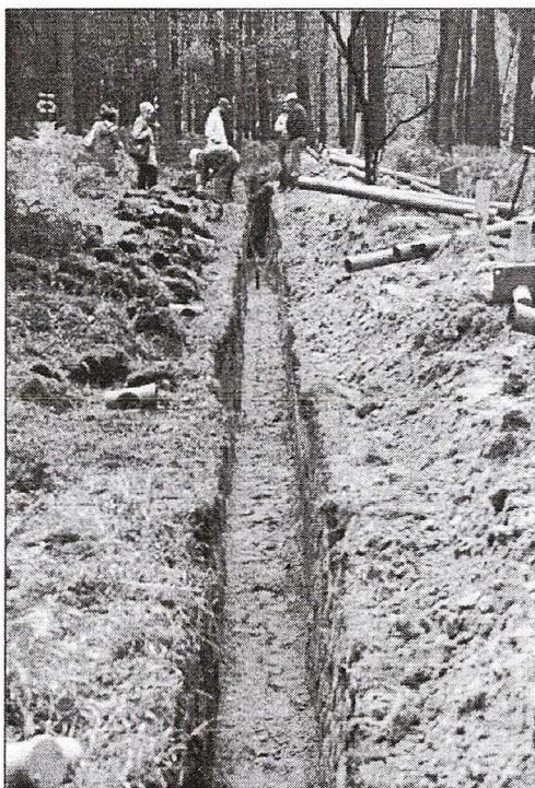
Fig. 4A. Trench for installing transducers
