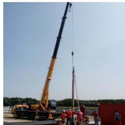
Fig. 16. Heater downhole procedure
