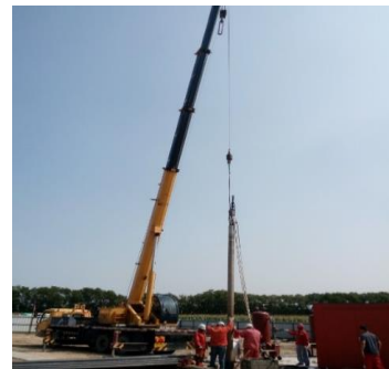
Fig.16. Heater downhole procedure
