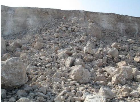
(a) Fragmentation of full-column charge holes after blasting at Bench-1
