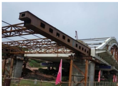
Fig. 1. The construction drawing for top-down construction of a steel truss arch bridge
