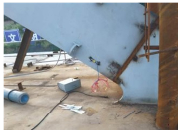
Fig. 9. Surface strain gauges on the arch rib
