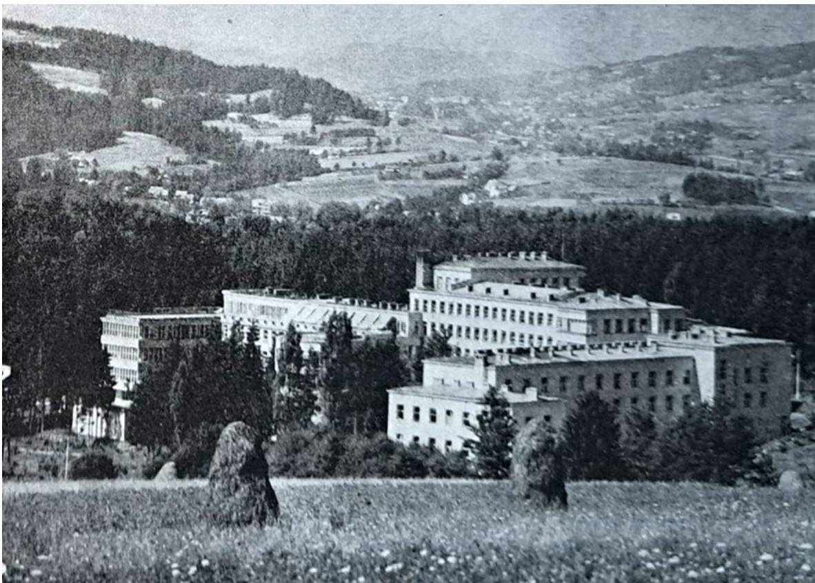
III. 4. Sanatorium GORD after the construction of the east and west wings of the building. Source: Ciechanowicz 1958.
