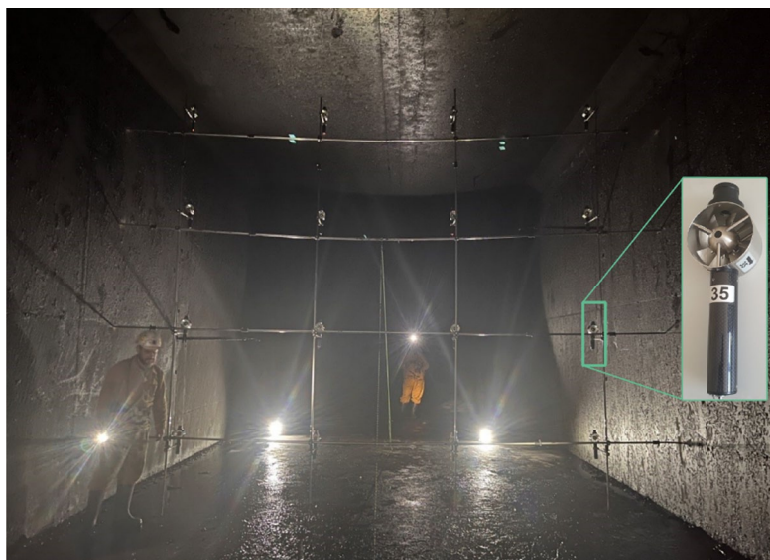
Photo 1. View of the measurement station in the collecting duct of shaft VI of the mine, enlarged view of SOM2303
