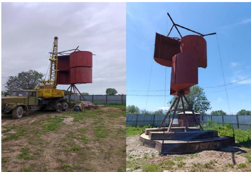
Fig. 8. Wind turbine assembly process
