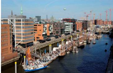
Fig. 3. The floating pontoon system of the Traditional Ship Harbour that raises and lowers with the tide offers moorings for more than 20 historic ships (original title). 13.11.2008
