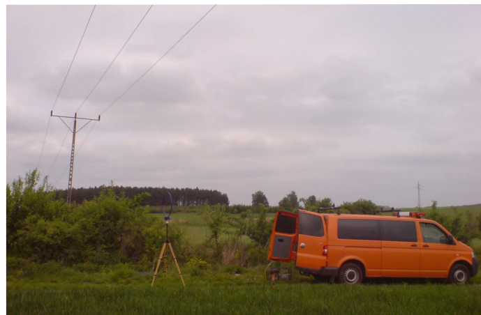
Fig. 14. Magnetic field measurement under overhead MV line
