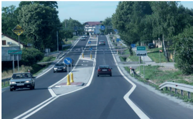
Fig. 1. View of the beginning of the model road section. Cross-section with additional multifunctional median lane.
